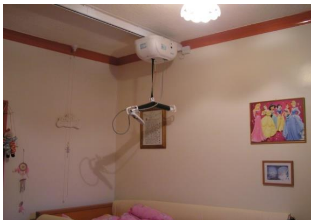
Ceiling Mounted Hoist
