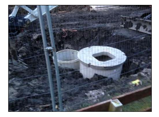
In line with Members' request, the case officer has queried the above with the applicant, who has clarified that the photograph shows standard concrete manhole rings (one for surface water and the other for foul water drainage) – they are not in fact tanks.
