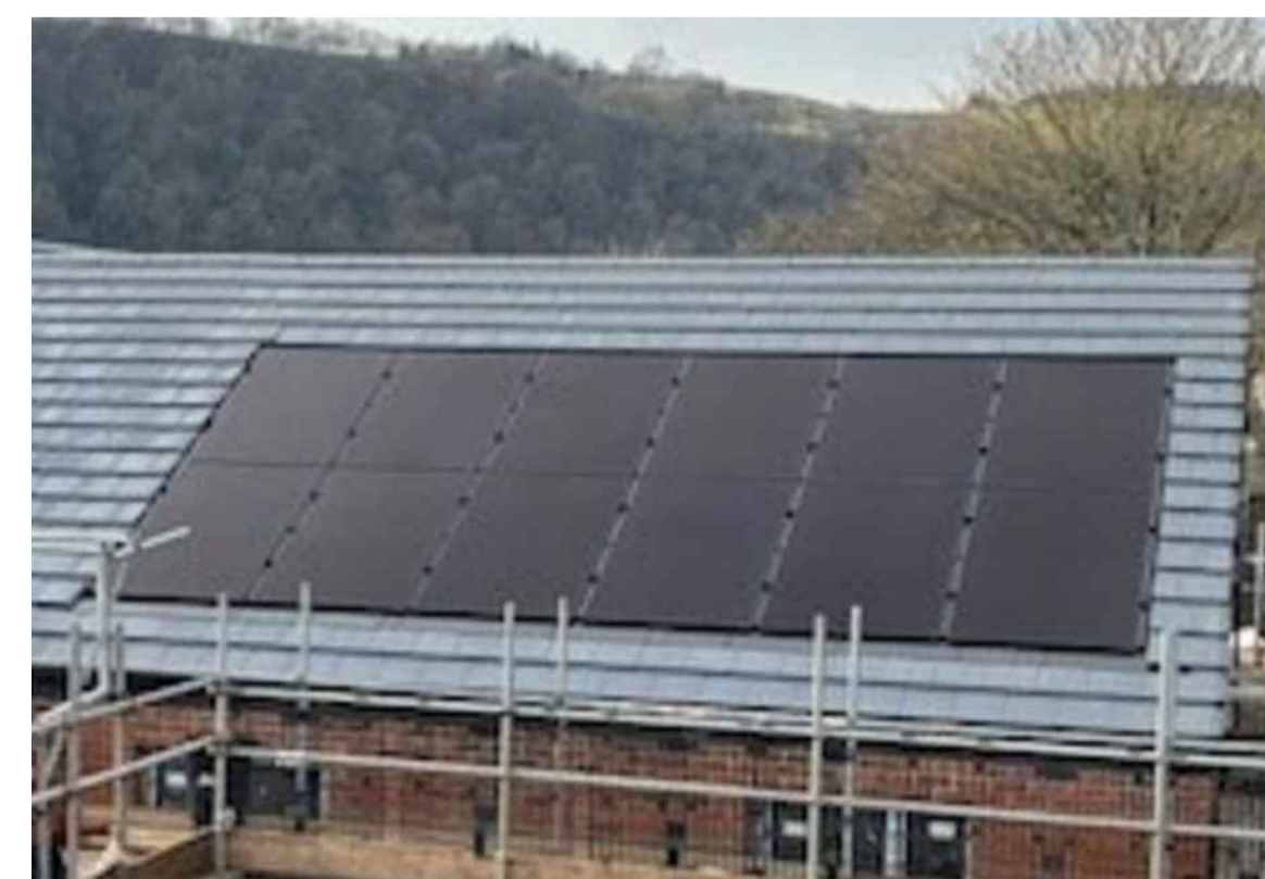
* typical 'inline' PV panel installation scale NTS
