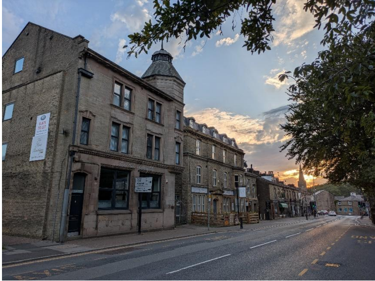
View from Bacup Road including the former Lancashire and Yorkshire Bank, The Royal Hotel and the Church of St James the Great
