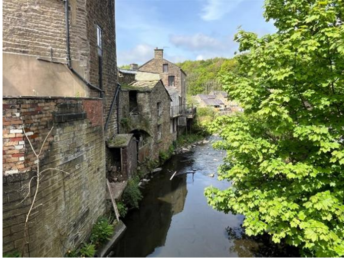
View of the River Irwell and buildings along Bacup Road
