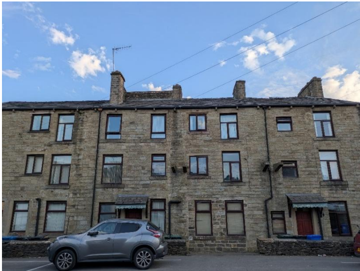
Three storey Stotts buildings
