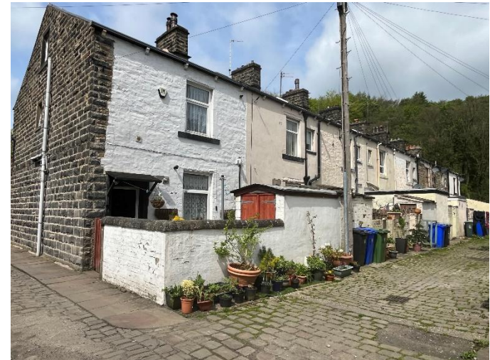
Rear elevations of 1-15 West Street
