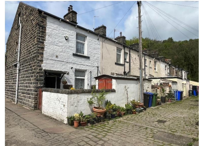
Rear elevations of 1-15 West Street
