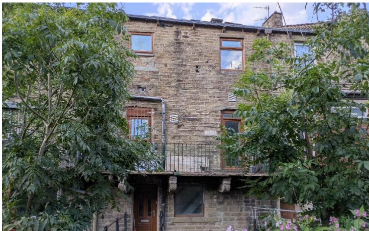
Shops/cottages along Bacup Road are two storey to the road and three storeys to the river with substantial stone balconies.
