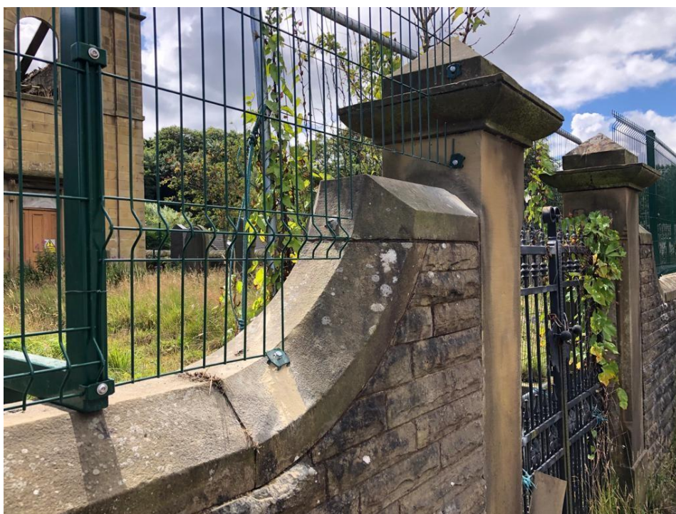
View of gates on Brandwood Road
