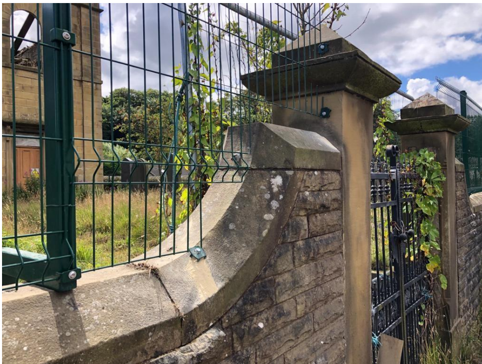
View of gates on Brandwood Road
