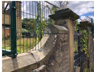
View of gates on Brandwood Road
