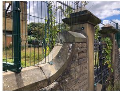
View of gates on Brandwood Road
