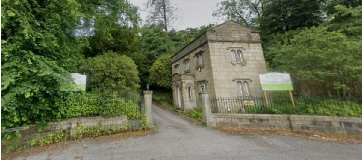
Plate view of the Entrance to Crawshaw Hall including listed Gate Piers and listed Gate Lodge
