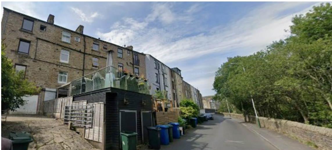
Station Road view (Rear of buildings 374 -406 Holcombe Road) Positive impact – low housing)
