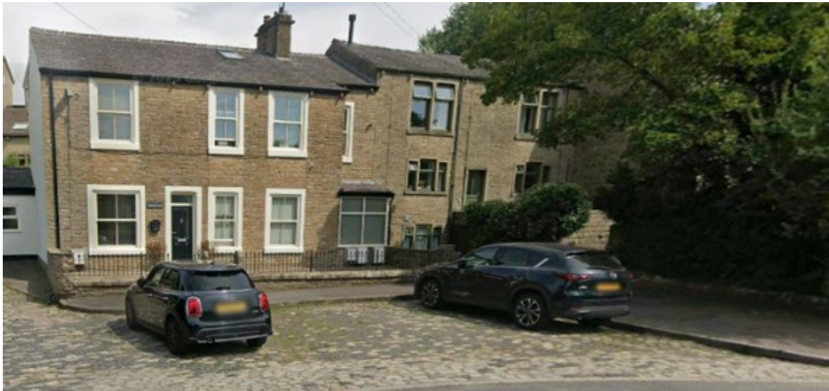
Nos 7 – 1 Bridge End (Positive impact – medium)
