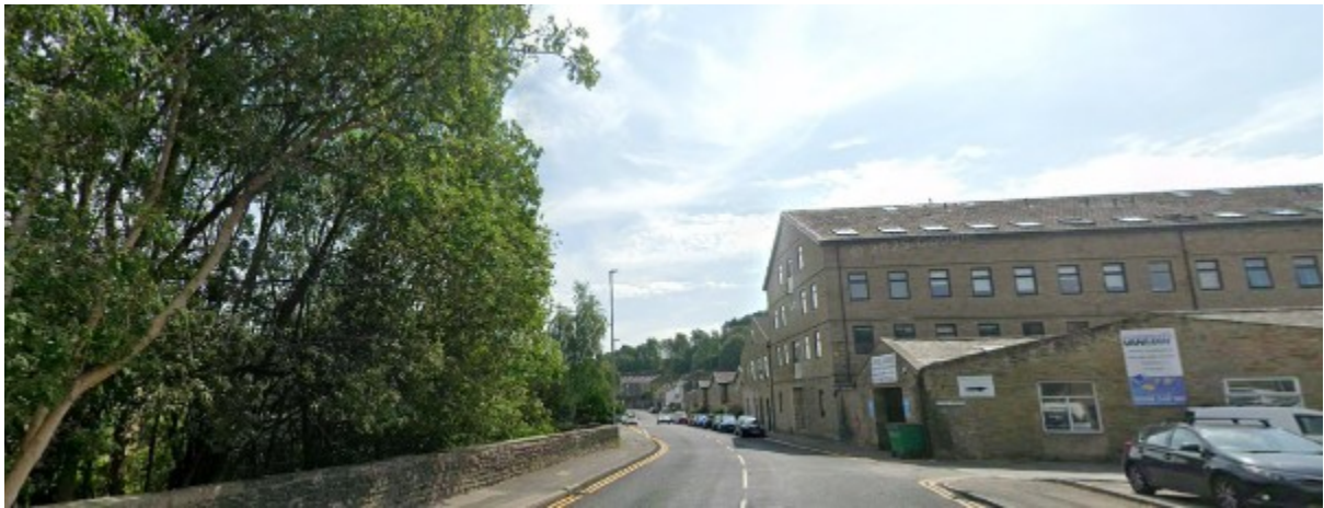
Looking south -Wavell House, Holcombe Road (east side) (Former Middle Mill) (Positive impact)
