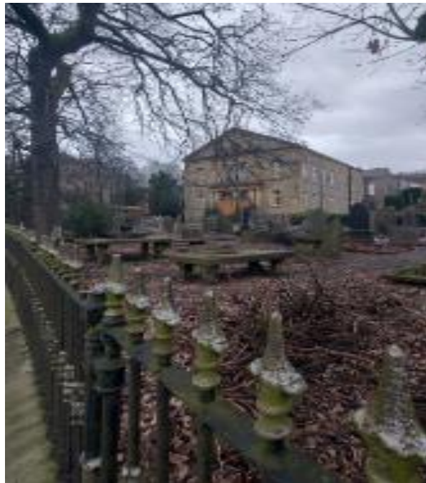
Plate Former Primitive Methodist Church and Sunday School, Lord Street
