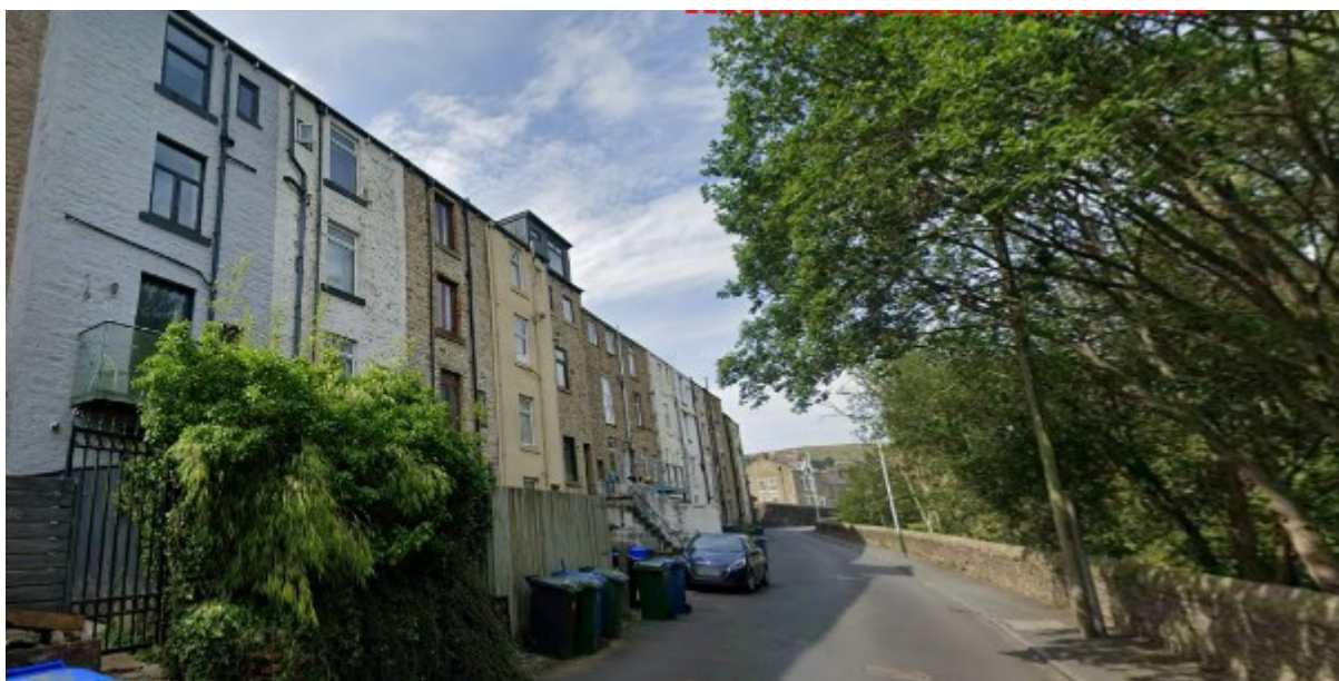
Station Road view (Rear of buildings 374 -406 Holcombe Road) (Positive impact -low)
