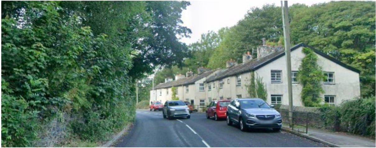
Looking North (Positive impact houses – high Listed Buildings)
