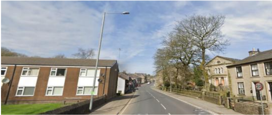
Plate view from Rake Foor Bridge including Nos 1-6 Kershaw Close and Nos 567-569 Burnley Road plus Rakefoot Methodist graveyard and church
