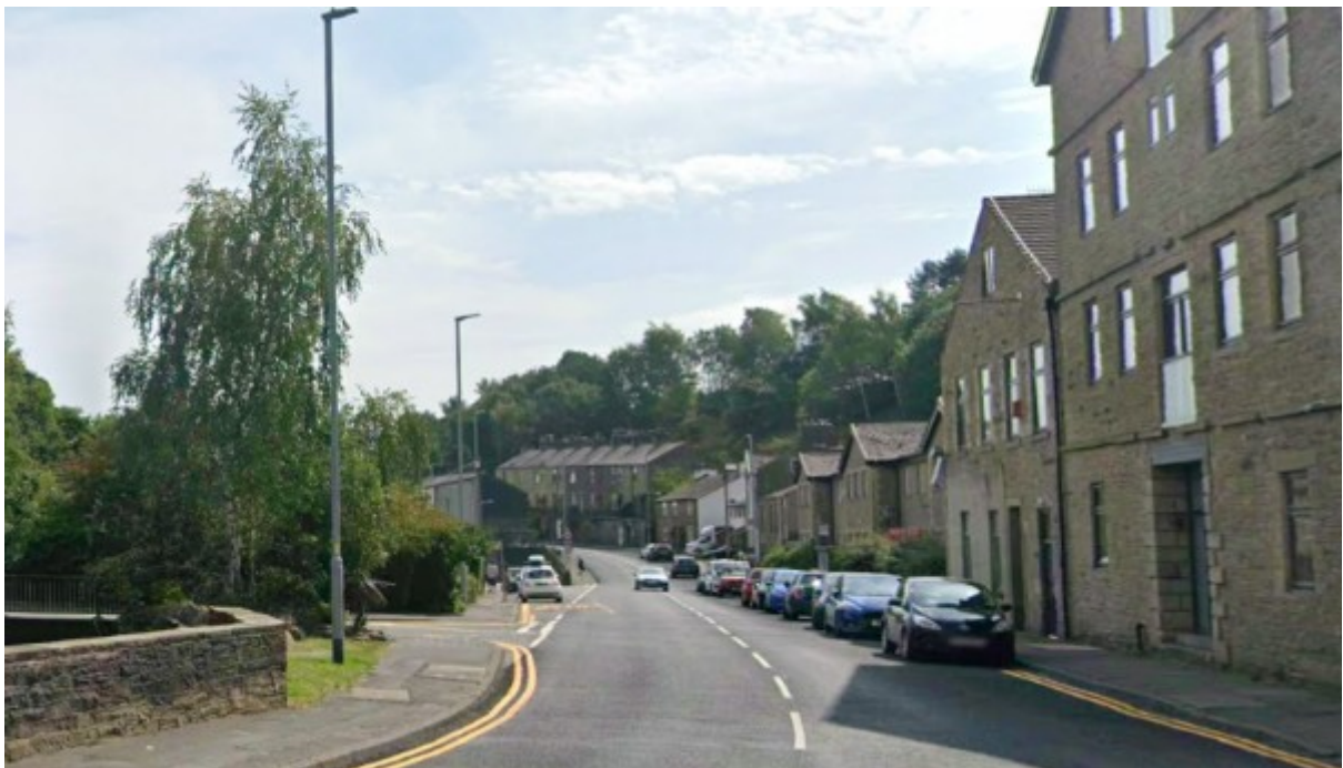
Looking south Wavell House Holcombe Road (west side) (former Middle Mill) (Positive impact)
