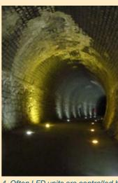
4. Often LED units are controlled by movement detectors switched on as the traveller passes through. This level of sophistication is probably not warranted on the relatively short tunnels here
