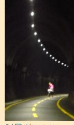
2. LED strips are more closely spaced resulting in an even lighting
