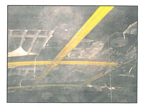
58 Ceiling collapse and steel exposure
