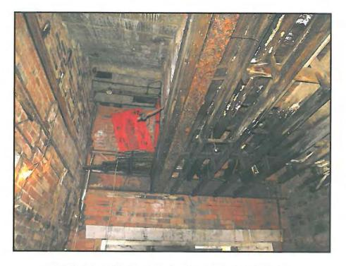
25 Entrance foyer - deterioration to steel and timber
