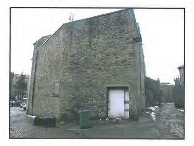
6.2 Weathering and deterioration is evident to the skew quoin stonework with joint losses in the order of 10 - 20 mm. (Photograph 15)
