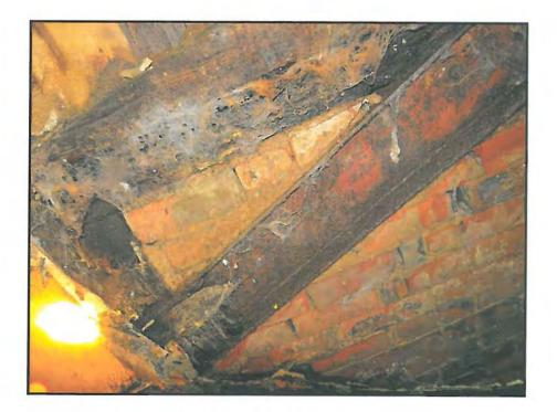
63 Steel corrosion and timber roof
