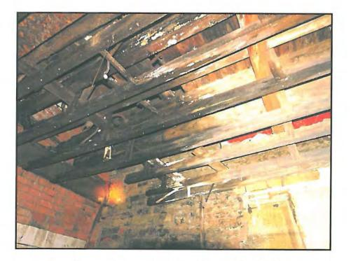
26 Entrance foyer - deterioration to steel and timber
