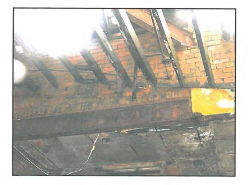
57 Roof collapse, rear (Southern) slope
