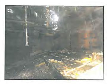
8.17 Some slating is evident on the rear Southern roof with deterioration to the main structural steelwork and continuing collapse of the rafter sub structure. (Photograph 57)
