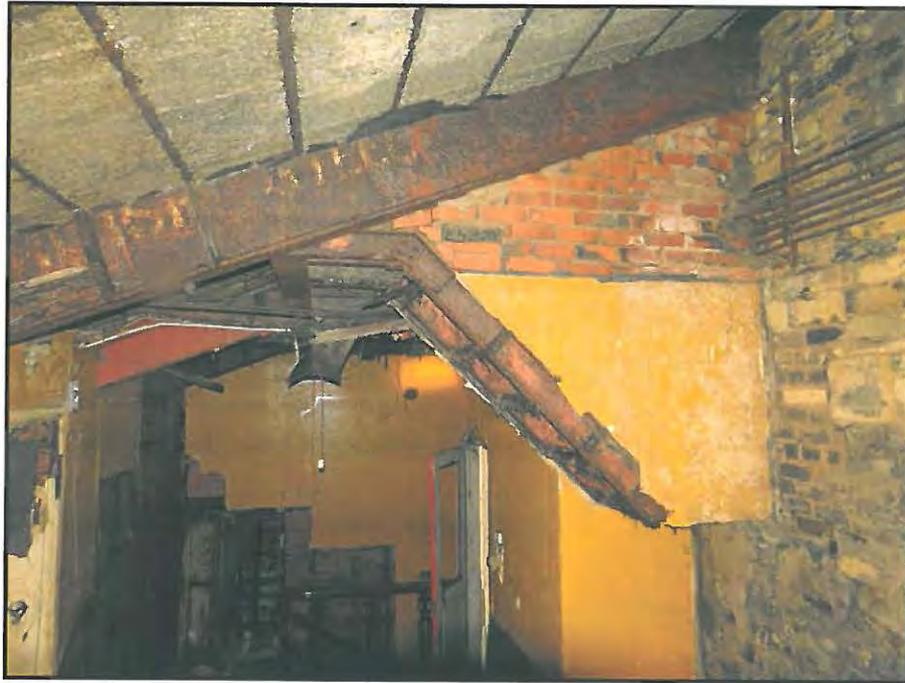
64 Steel corrosion and timber roof
