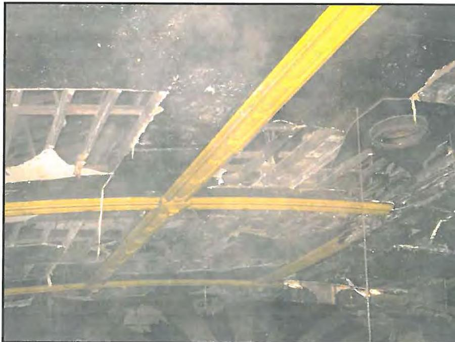
58 Ceiling collapse and steel exposure
