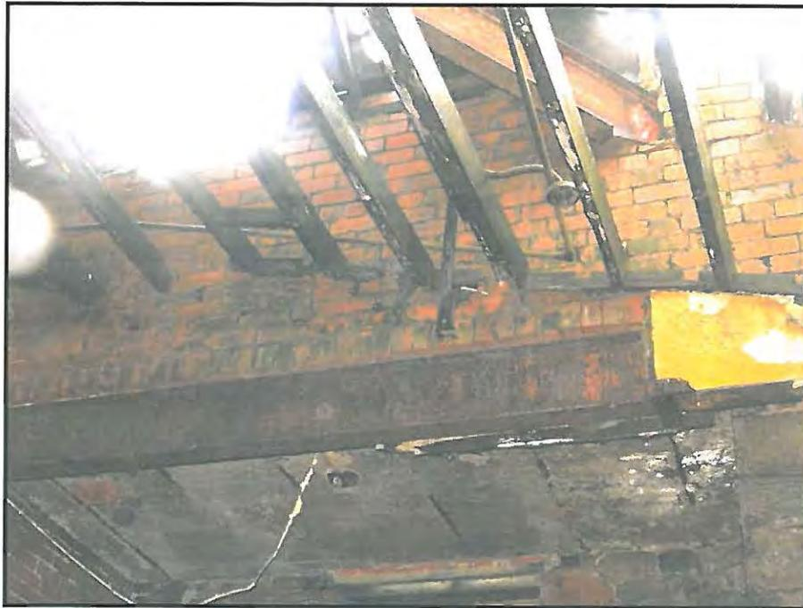
57 Roof collapse, rear (Southern) slope
