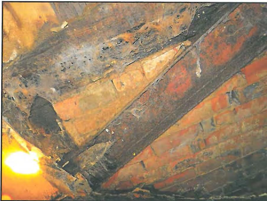
63 Steel corrosion and timber roof
