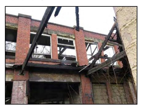
11.12 At first floor level on the main unit (Unit 4) severe spalling is evident to all the concrete lintels at first floor level to Bays 1-4 with spalling of the concrete and exposure of the main reinforcement. (Photographs 081, 082, 083 - close up).
