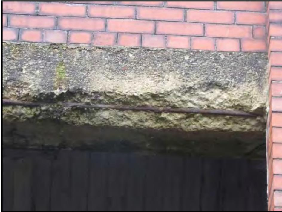
083 Typical spalling to concrete lintel, Unit 4
