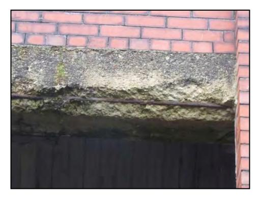
083 Typical spalling to concrete lintel, Unit 4
