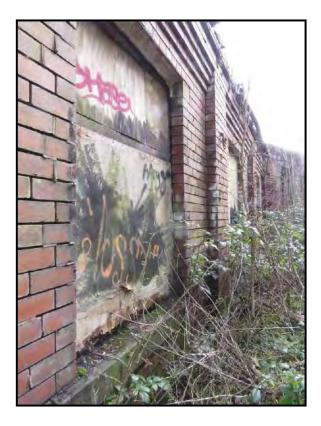
7.5 The rear North Western wall to Unit 3 extends for a further 30 metres with a 2 metre square opening flanked on the right hand side (South West) by two Bays between brickwork piers incorporating rectangular windows on stone cills beneath a four course deep corbelled brickwork head. (Photographs 034, 035).
