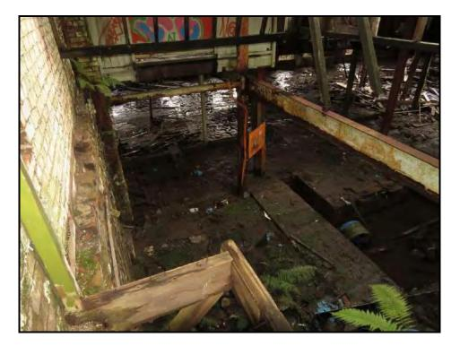
044 Collapsed first floor Unit 6 to ground floor Unit 6
