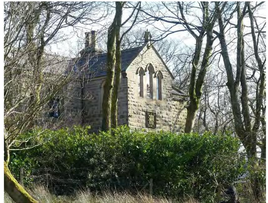
4.37 The eastern elevation backs immediately onto Goodshaw Lane with a former entrance that appears to have been partly infilled and converted into a window and an unusual Romanesque round arched first floor window with a zigzag moulding supported by slender columns.
