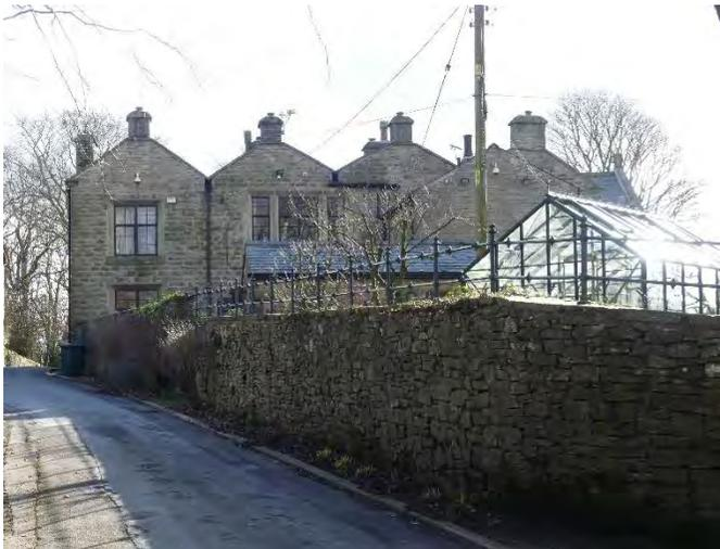
4.36 The entrance wing contrasts with the rest of the composition by projecting at right-angles from the western gabled range. The detailing is contrasts, including three lancet windows to the first floor above the main entrance and single lancets to the side elevations.
