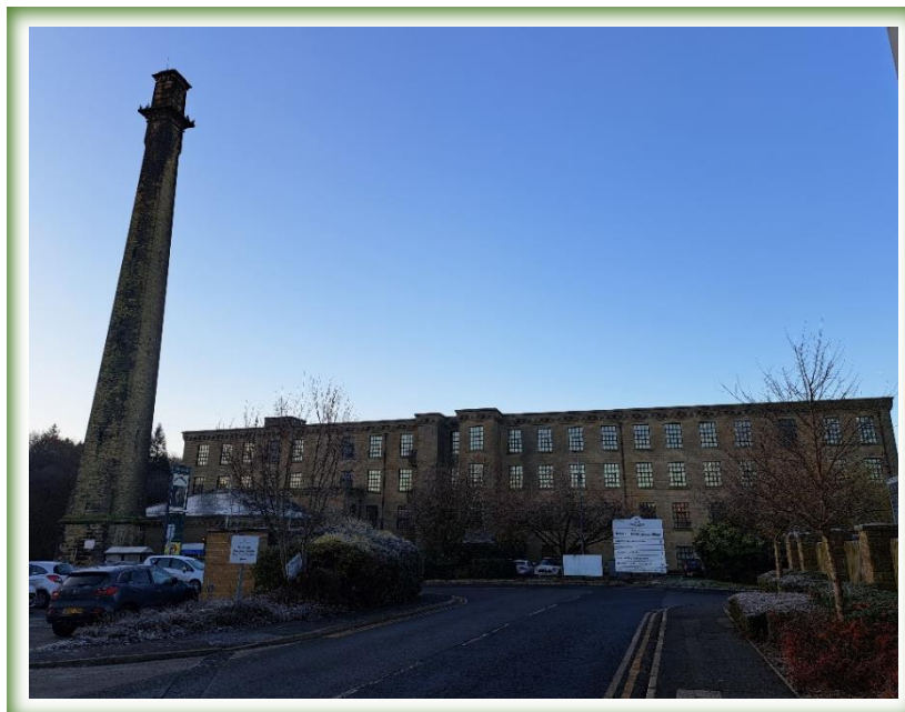
Figure 2- Hardman Mill, New Hall Hey. Source: Forward Planning, Rossendale Borough Council
