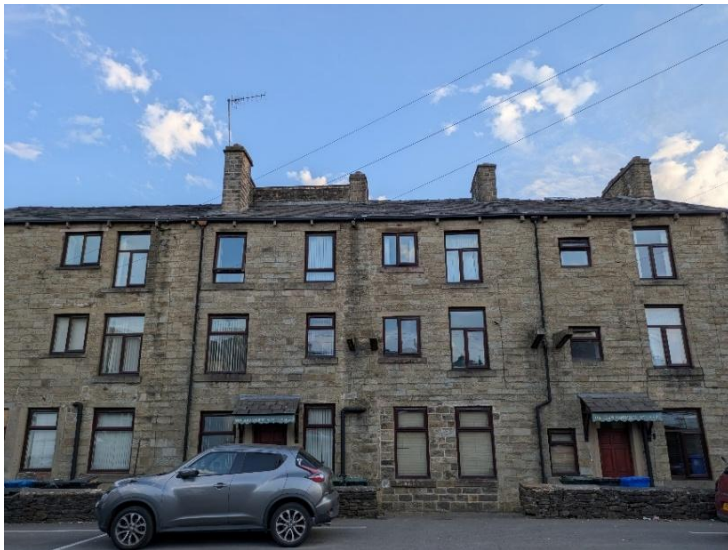
Three storey Stotts buildings
