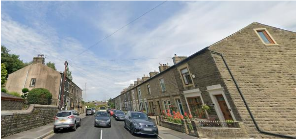
Nos 374 -406 Holcombe Road (east side)(looking north Positive impact -low including housing and wall)
