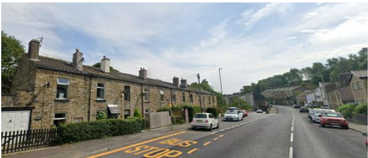
Looking south -Nos 352 – 374 Holcombe Road (east side) (Positive impact – Medium)
