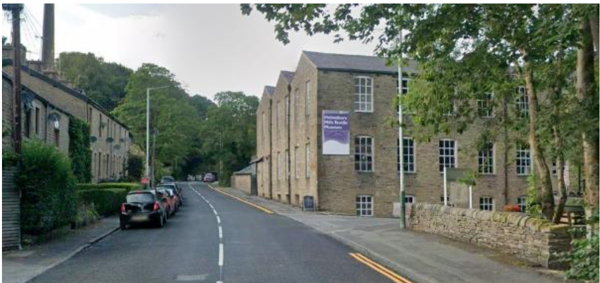
Looking north - Nos 287 – 271 Holcombe Road (west side) Higher Mill and Helmshore Mill Museum (east side) (Positive impact high- Mills, medium - walls and low housing)
