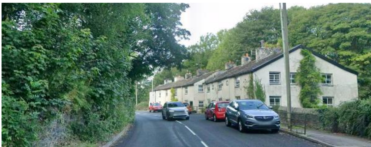
Looking North (Positive impact houses – high Listed Buildings)
