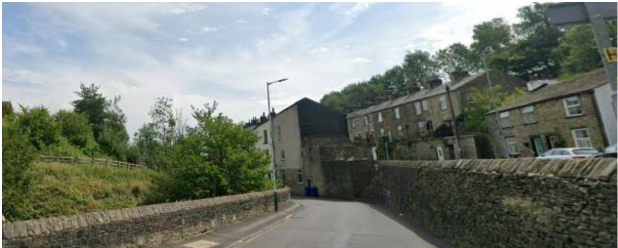
Looking south- Station Road with River Ogden (east side) (Positive impact – low)
