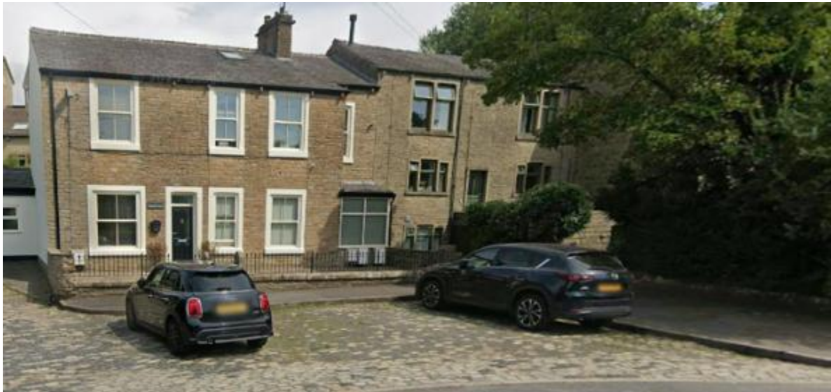
Nos 7 – 1 Bridge End (Positive impact – medium)
