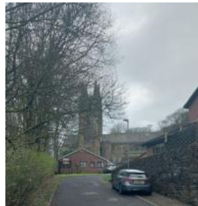
Plate Rakefoot Bridge over Limy Water (within CA) with modern dwellings(outside CA)
