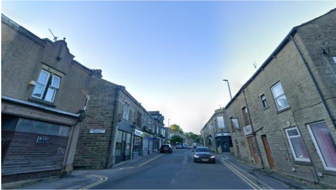
Plate looking north along Burnley Road with traditional shopfronts evident Nos 570-586 on left
